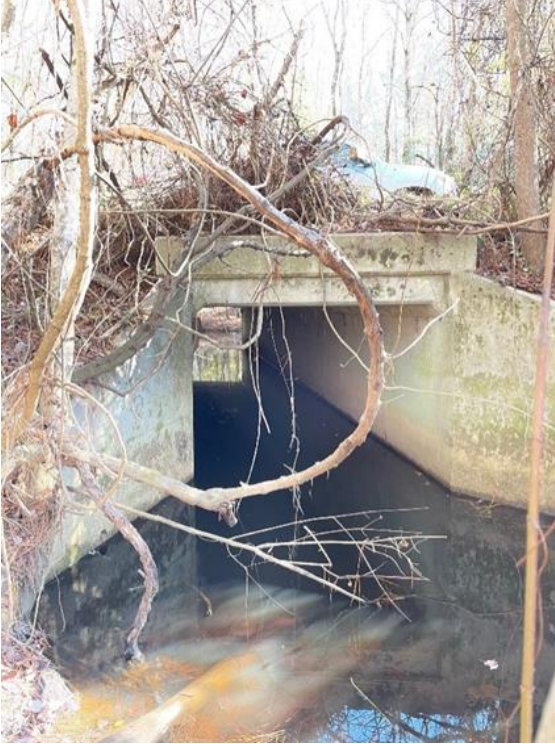
Culvert 4 (Sta 119+25) US Inlet
