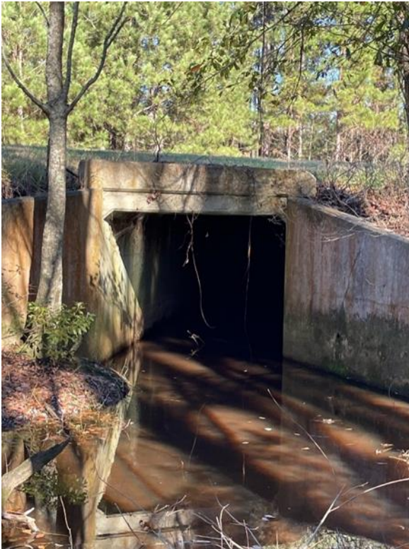
Culvert 3 (Sta 3214+28) US Inlet
